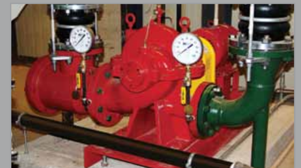
East Hartford High School —EnviroFlo Horizontal Split Case Pumps met critical construction schedule demands with easy, groutless base installation. Now they're providing high efficiency primary/secondary chilled water and condenser water movement for reliable student/teacher comfort.
