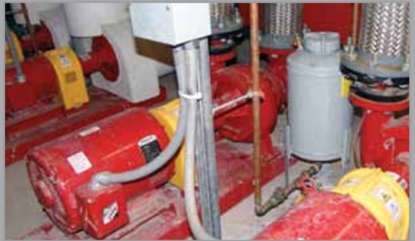
Rhode Island School of Design—EnviroFlo Frame-Mounted End Suction and Vertical In-Line Pumps are maintaining critical climate control requirements in a 128-year-old library while minimizing energy consumption.
